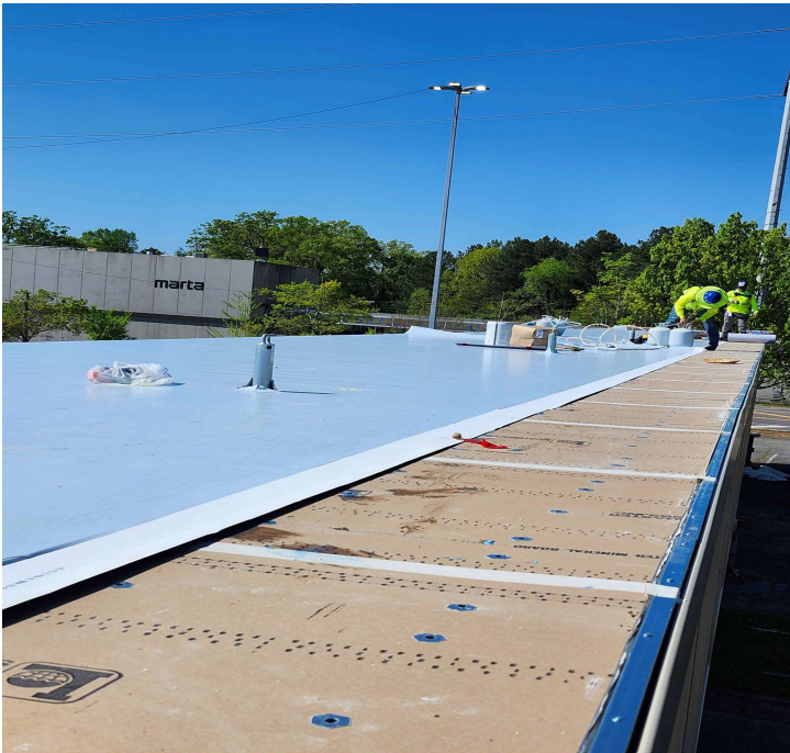
Install of Single-Ply Membrane
