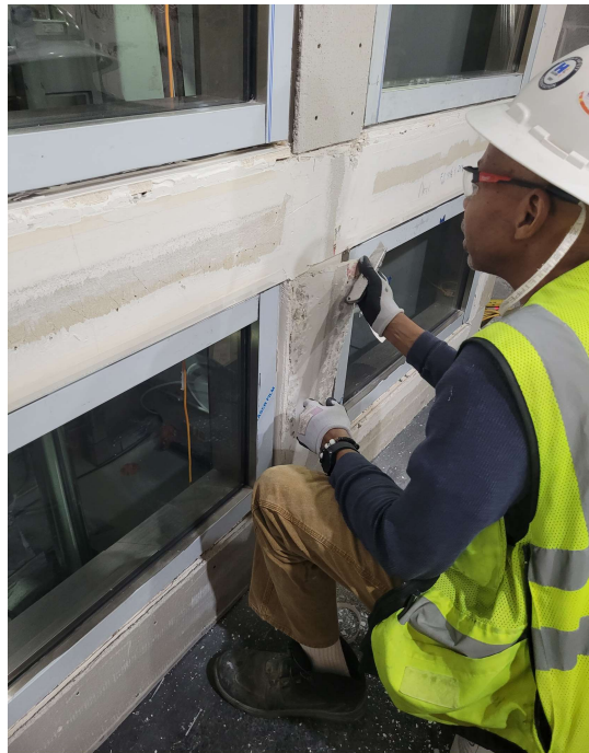
Sheetrocking the window frame
